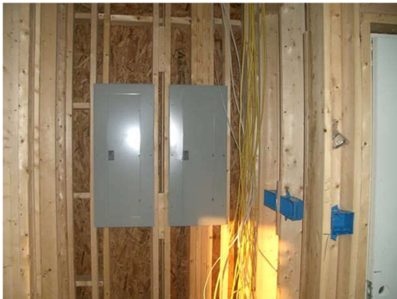
Two 400 amp breaker panels being installed
