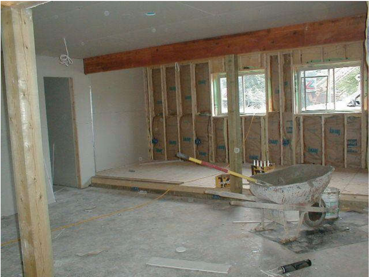
Construction of Luna City 1.0
