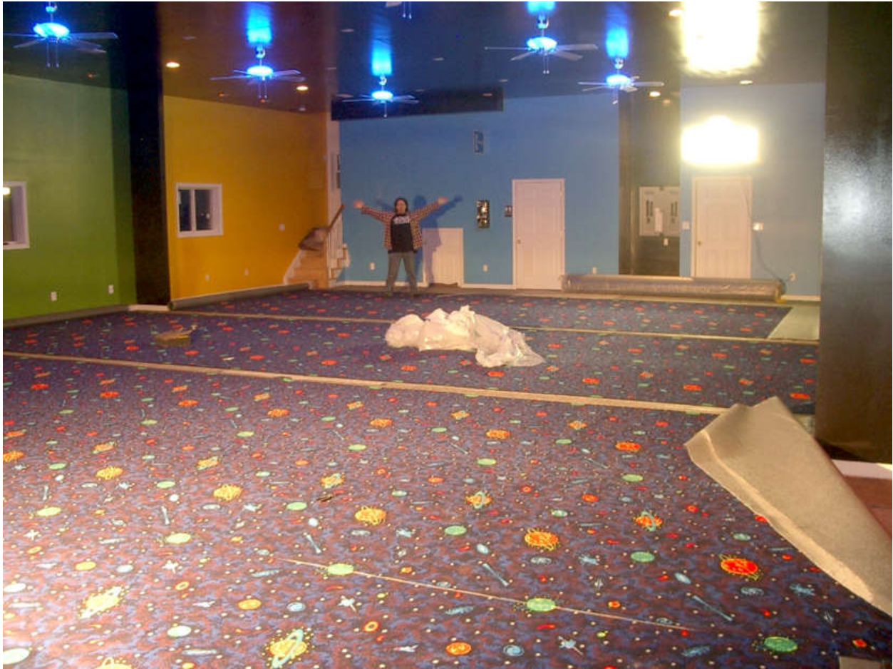
The new blacklight carpet being installed!
